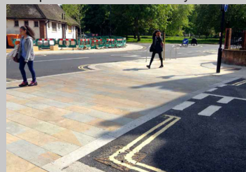
Example of continuous footway
